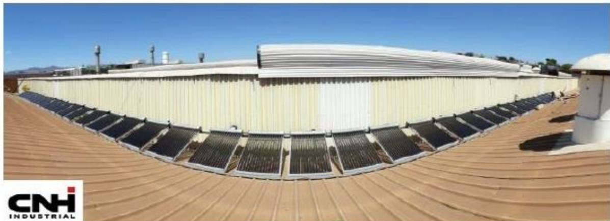
Figura 13 – Coletor Tubo Evacuado Modular All-Glass (TEMAG)
